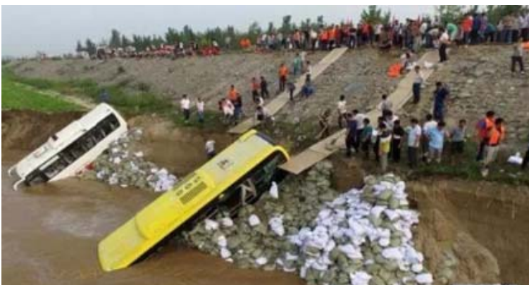
Repairing the river bank with scrapped buses Xingtai, Hebei July 23, 2016 (People's Daily)
